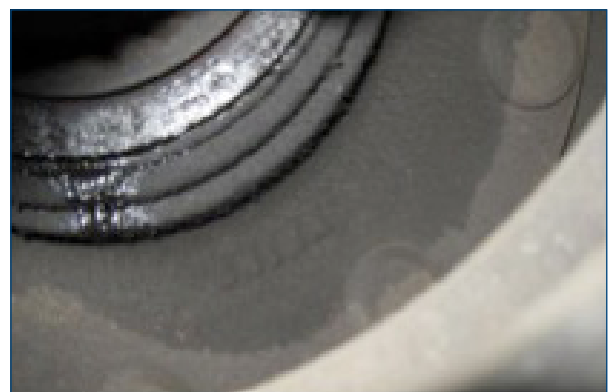
FIGURE 4: Leaking - Change Seal
