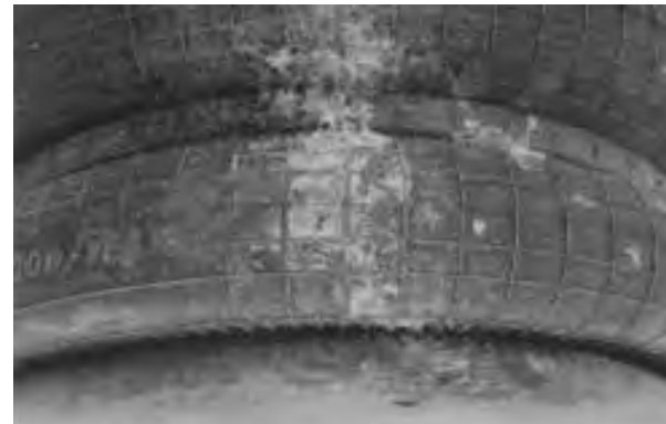
DAMAGE FROM CHEMICALS
