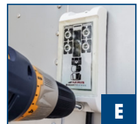
Example of using a pop rivet to install the bracket.
